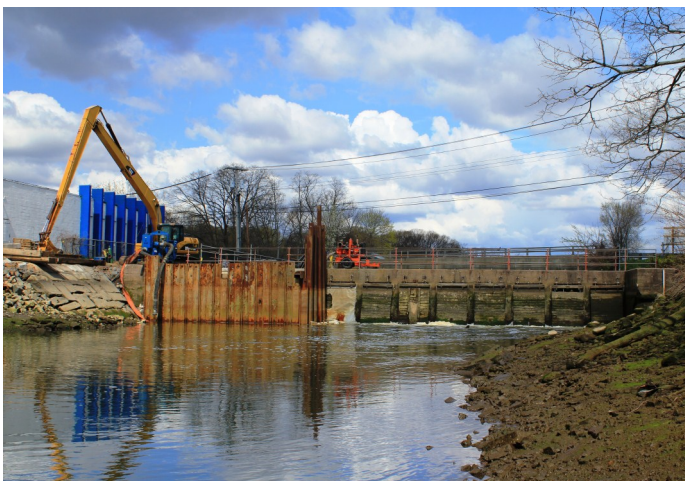
Tide Gate Construction, April 2012
