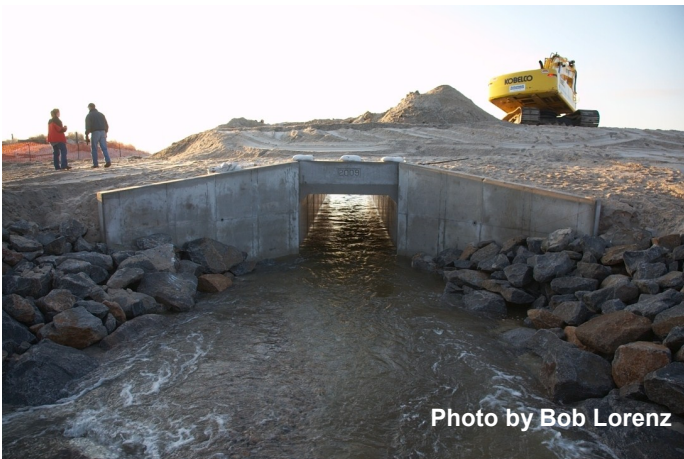
Culvert Construction, January 2010
