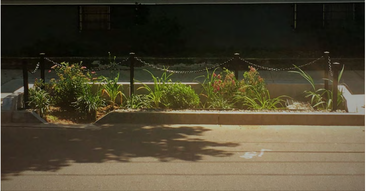
Figure 9. (above) Bioswale installed in the City of New Haven. Credit: Dawn Henning, City of New Haven Engineering
