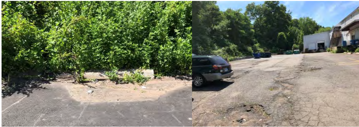
Figure 21. Existing conditions at Counter Weight Brewery, showing clogged catch basin (left) and degraded asphalt parking lot (right).
