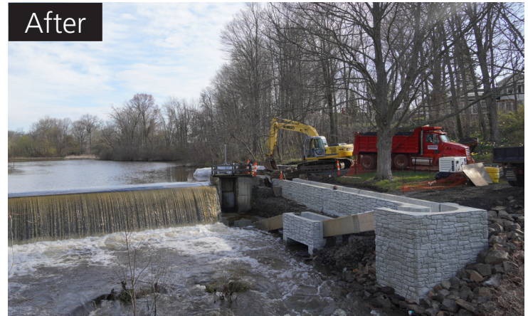
The new fishway allows migratory fish like Alewife to climb up and over the dam using a series of ramps outfitted with features to slow the velocity of the water and areas that allow the fish to rest.
