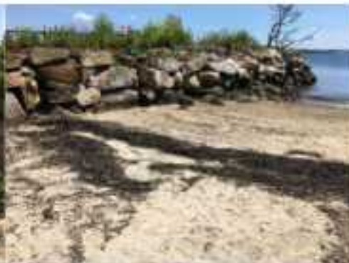
Closer overview shot of station Y.
