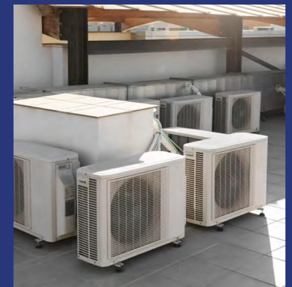
Packaged Rooftop Unit (RTU)
