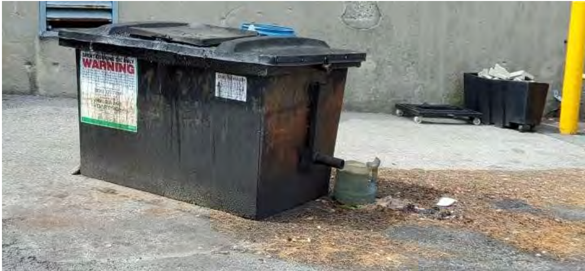
Figure 18. Hutchinson River Watershed Hotspot: Overflowing and Undermaintained Oil and Grease Disposal Container (Eastchester)
