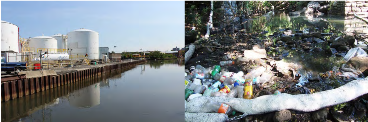
Figure 6. Petroleum Storage Tanks by the Eastchester Creek Channel (Mount Vernon) (left). Built-up of Litter in the Hutchinson River Behind Homes on Beechwood and Farrell Ave (Pelham) (right)
