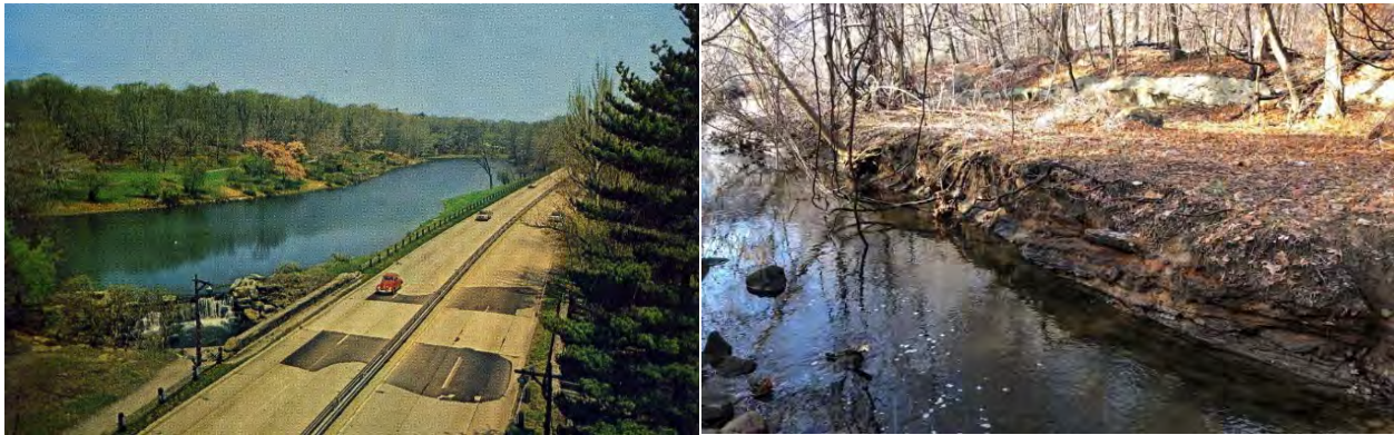
Figure 5. 1950s North Facing Postcard View of Pelham Lake (Mount Vernon) (left). Stream Bank Erosion along the Hutchinson River (right)
