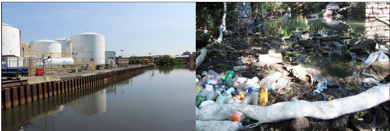
Figure 6. Petroleum storage tanks by the Eastchester Canal in Mt. Vernon (left). Built-up of litter and the polluted Hutchinson River behind homes on Beechwood and Farrell Ave in Pelham (right).
