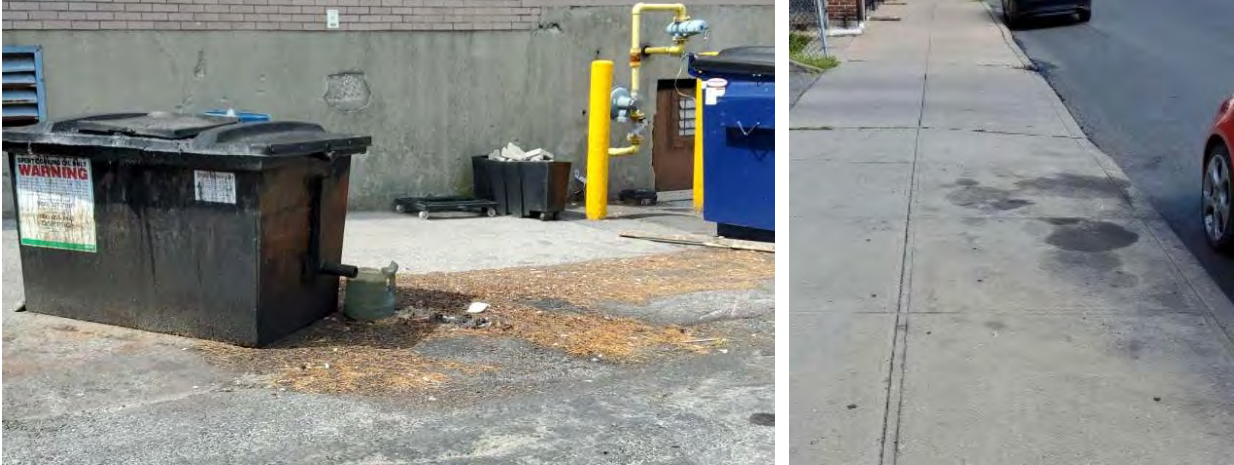
Figure 7. Large Grease Stains along Pavement
