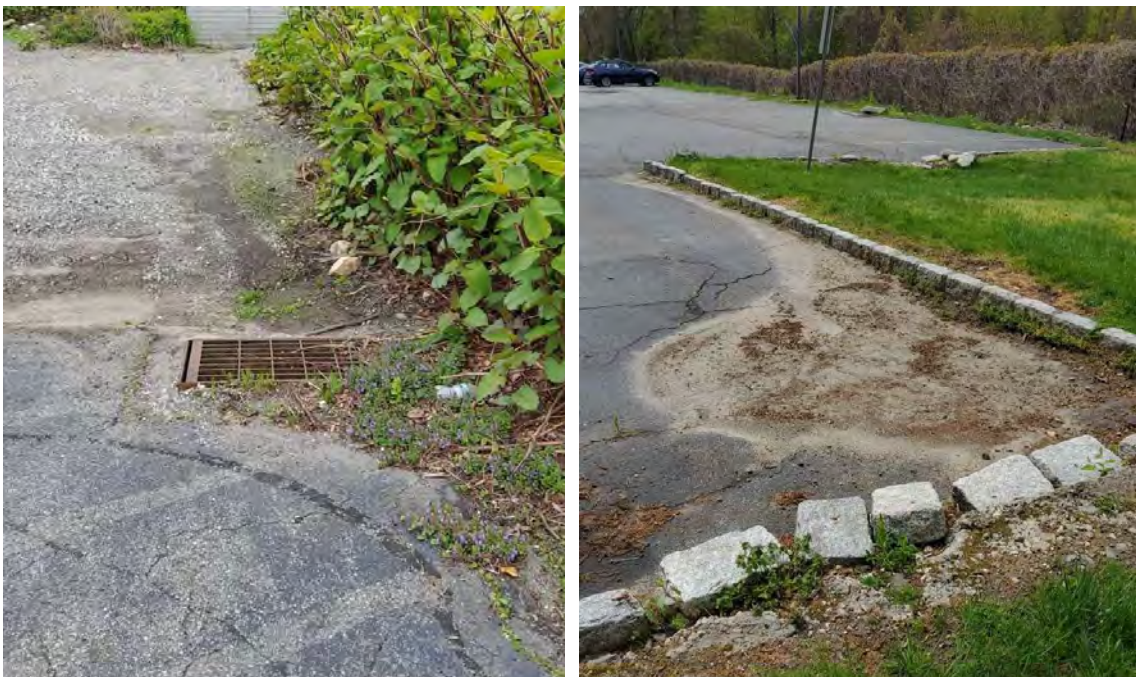
Figure 12. Locations with Evidence of Ponding Pose Good Opportunities for Bioretention
